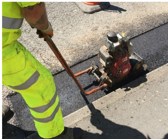
Figure 4 – Patch Repair of Pothole Style Defect
